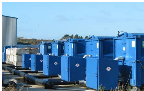
Fig.2. The In-vessel composting system at Kilbarry. In-vessel containers, aeration cabinets, manifold piping and the biofilter are illustrated.
